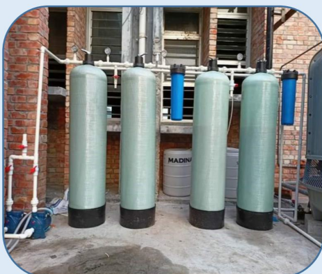
Installation of WTP for an Industrial Building.
