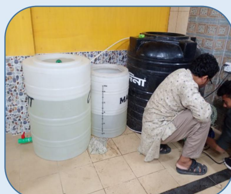
Installation of Disinfection Plant for Hospital Project.
