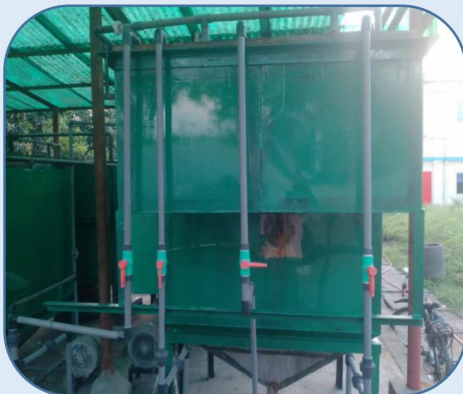
Installation of ETP for Textile Industry.
